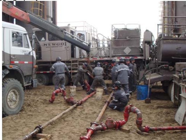
Rigging up Hydraulic Fracture Stimulation in Western Siberia
